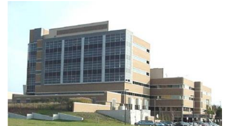
Victoria Research Laboratories at Victoria Hospital, home of the Baines Centre
